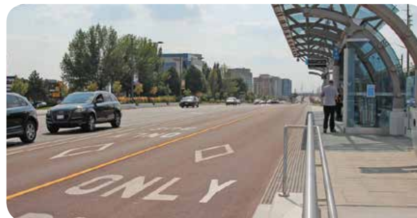
Median Running BRT in Suburban Area
