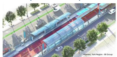
A median station is located in the median of a centre of the roadway at intersections for a median running way or bus lanes.
