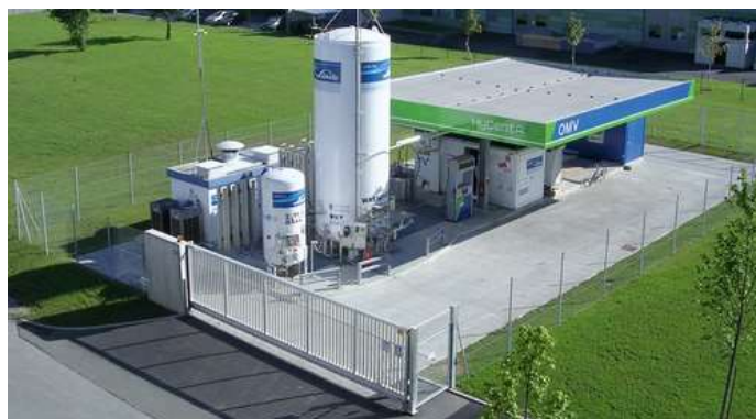
Figure 35: Linde fill station - liquid hydrogen delivery, on-site storage and dispenser model. Source: adapted from [104]
